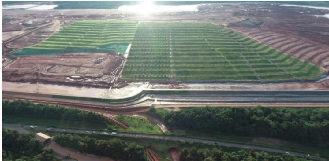
Figure 10. General View – DRS1 Reclamation, Hydro Alunorte.
